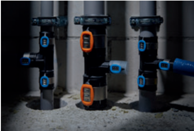
STRIKING PRESSING INDICATOR Even in difficult visibility conditions, it is still clear to see whether the pressing indicator is still on the fitting or the connection already pressed.
